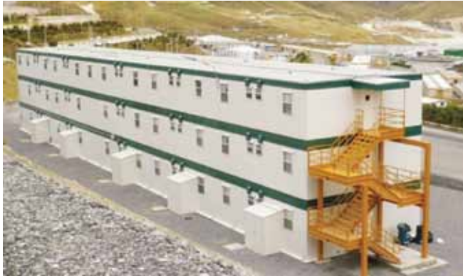
Housing units in Antamina built for miners that live at 3800 metres above sea level or more.
