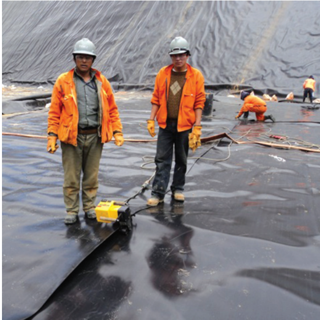
El Aliso workers installing liner materials at Yanacocha. (Photo courtesy of El Aliso)
